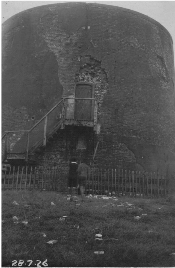
Damage to the tower
